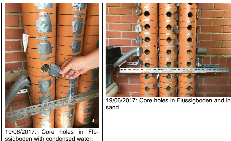
Figure 23: Continuation of the test until 19 June 2017 with sealed holes
